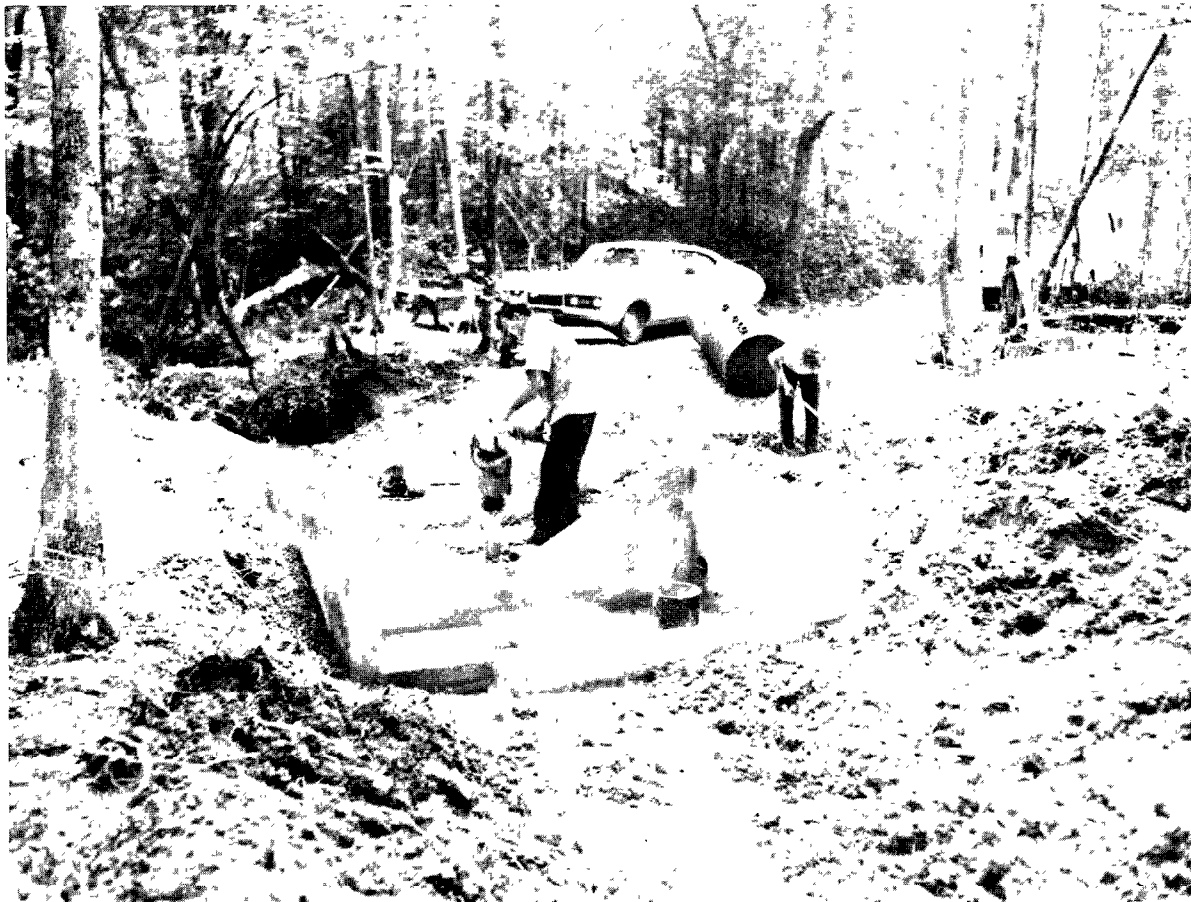
FIGURE 31.—Vertical support walls and energy-dissipation box at early stage of construction of 1-foot trapezoidal supercritical-flow flume.
